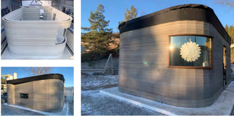
Figure 2.10: A 24 m 2 house demonstrator project was the first 3D printed building in Sweden by ConcretePrint [92].
