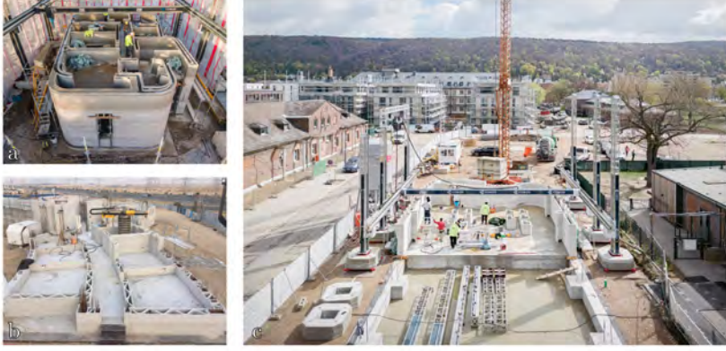
Figure 2.7: Examples of 3DCP projects with on-site printing. Left: Beckum House [44]. Centre: Municipal building in Dubai [85]. Right: Data centre in Heidelberg.
