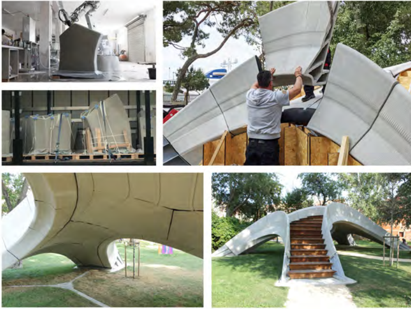
Figure 2.14: The manufacturing, transport, and assembly of the Striatum Bridge. Images from [16]
