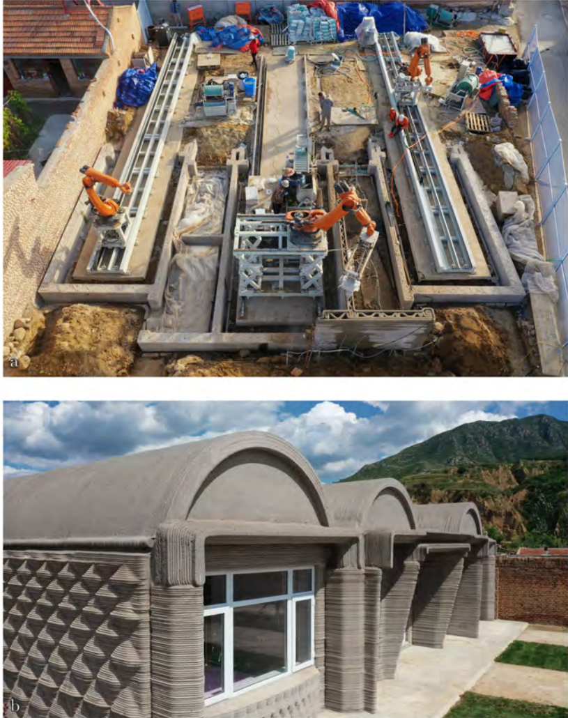
Figure 2.8: The Wujizhuang farmhouse featured three tracks for the deployment of the 3DCP system based on robotic arms. The different orientations used for printing roofs are visible in the ribbed surface of the structure. Reproduced from [89]
