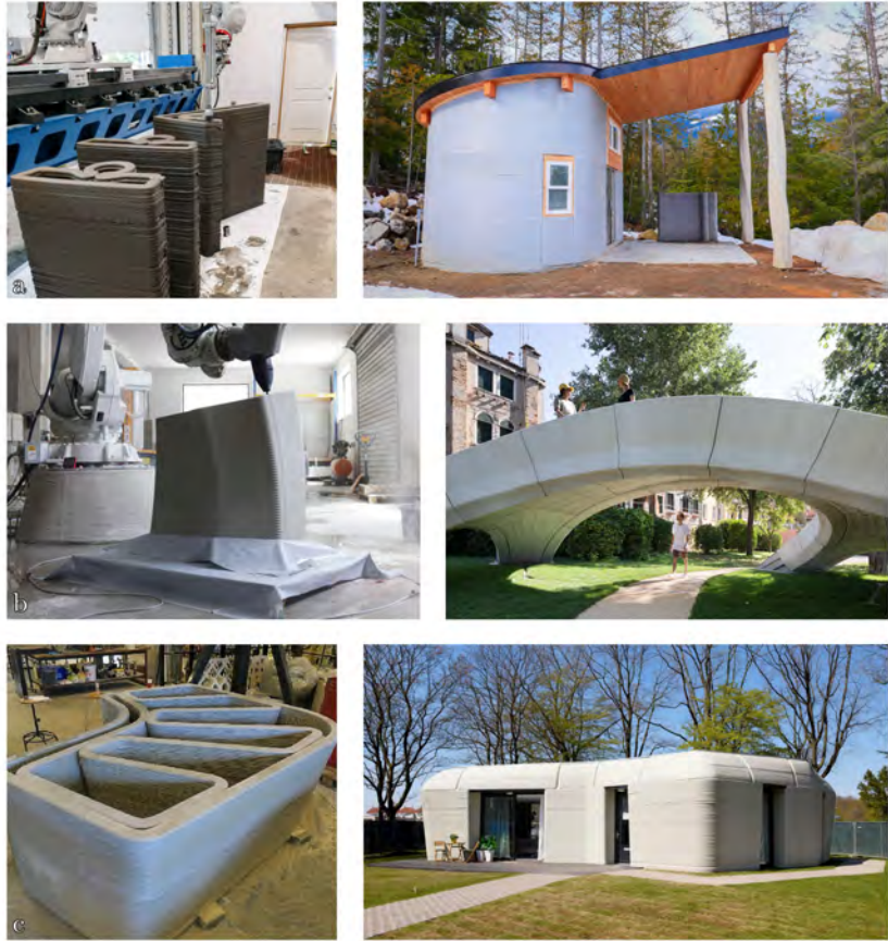
Figure 2.6: Examples of 3DCP projects printed as prefabricated elements and assembled on-site. Top: Fibonacci House, Canada. Middle: Striatum Bridge, Venice. Bottom: Milestone project, Eindhoven.
